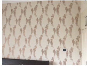
Walls and ceiling
