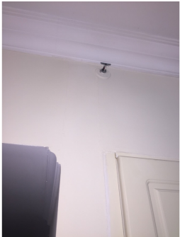
Walls and ceiling
