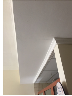
Walls and ceiling
