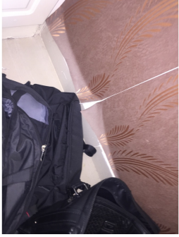
Walls and ceiling
