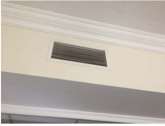
Walls and ceiling
